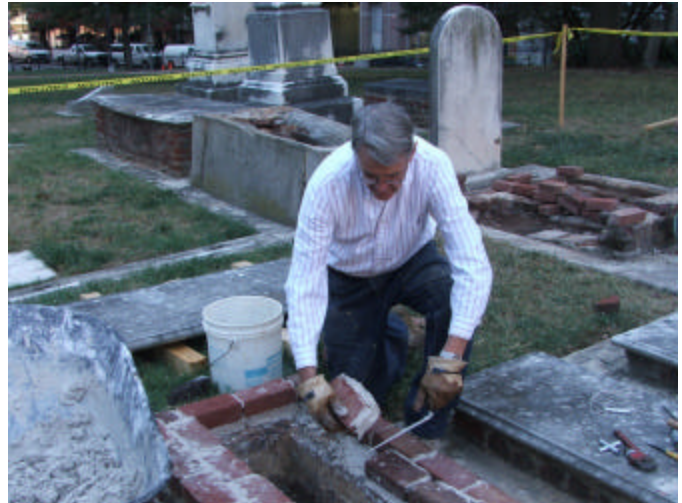
Jim Williams laying brick
