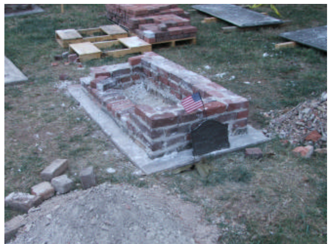
Brick box under construction
