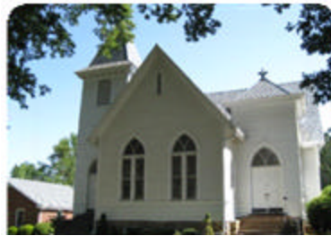
BANKS PRESBYTERIAN CHURCH 10012 New Town Road
